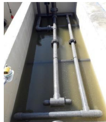
Figure 5 Submerged SiC membranes into existing settling tank
